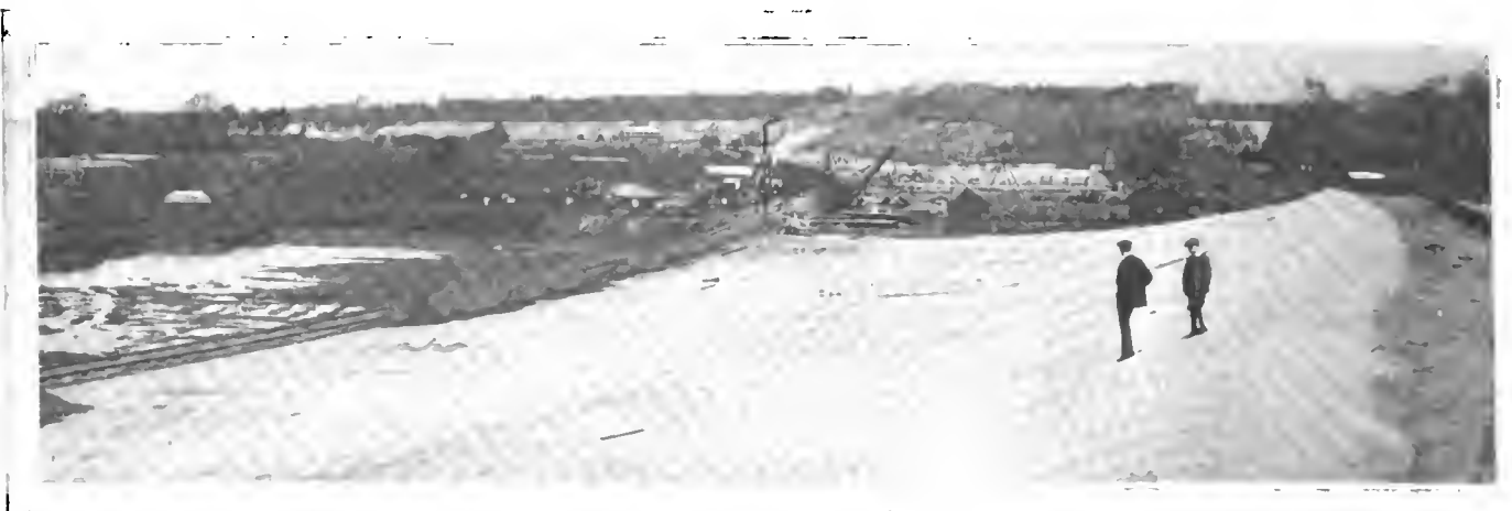
GENERAL VIEW OF BROOKLANDS AUTOMOBILE TRACK NEAR LONDON, SHOWING ONE OF THE BANKED CURVES FOR 100 MILE SPEEDS.
